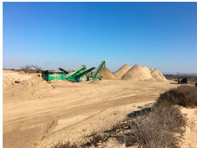
Cleared and processed sediment from the basin being prepared for transport off site.
