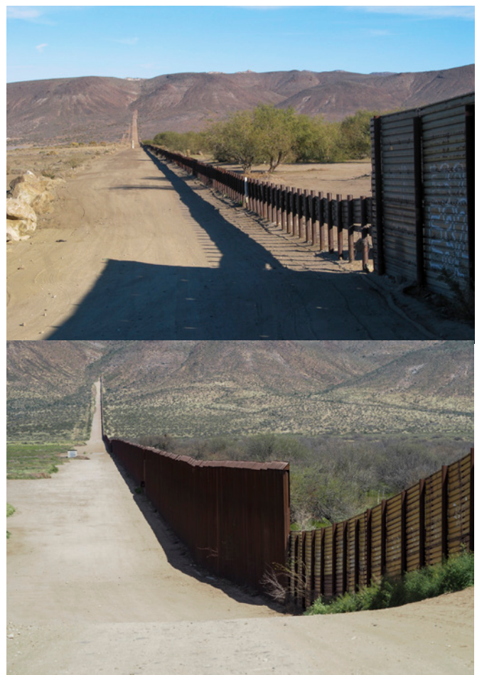
Border fence near Jacumba in eastern San Diego County. The image from 2002 (above) shows the 8-foot fence constructed from surplus landing mats and then a vehicle barrier in the valley bottom. The 2017 image (below) shows how the vehicle barrier was replaced with a pedestrian fence approximately 20 feet in height that also includes gates that open to accommodate stormwater flow and decrease flooding impacts.
