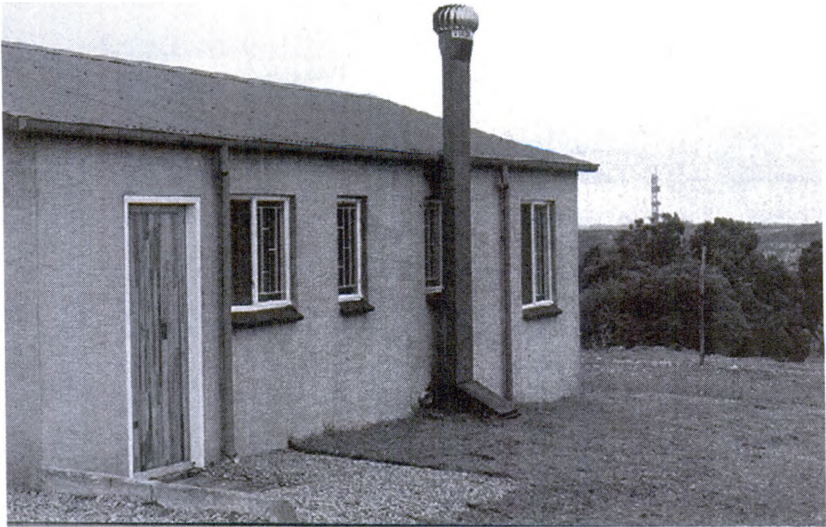
Figure 3: A Residential Installation of a Completely Enclosed Solar Latrine (Waterless)
